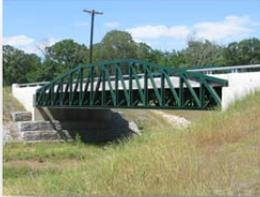
Prepared Engineering construction documents for an 80-foot span vehicular bridge. The hydrological/hydraulic aspects included preparing a FEMA Conditional Letter of Map Revision (CLOMR) and a Letter of Map Revision (LOMR) associated with the construction of the new bridge.
